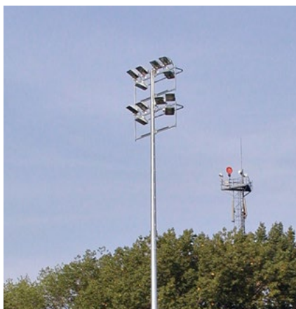
Fixed mast with ladder and twin platform
