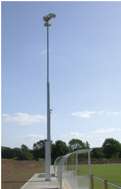
15m telescopic masts at Stone Dominoes Football Club in the UK. The local Planning department permitted a maximum permanent height of 8m.
