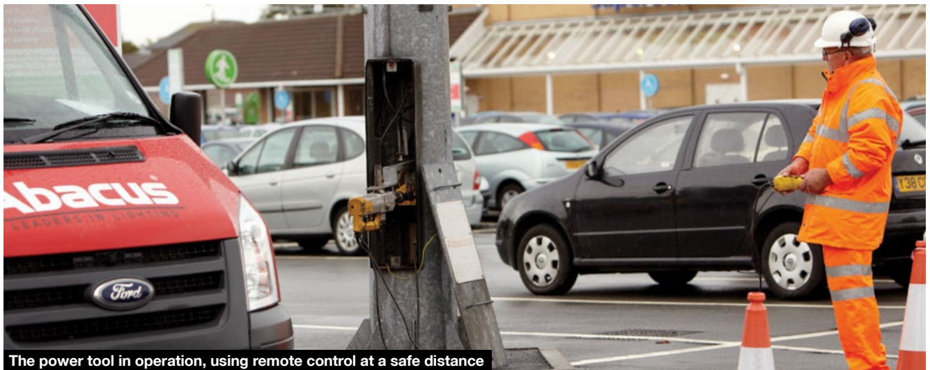
The power tool in operation, using remote control at a safe distance
