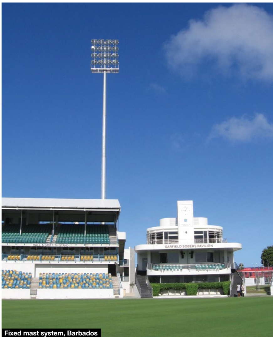
Fixed mast system, Barbados
